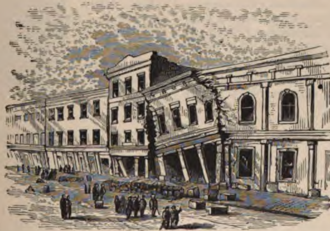
EARTHQUAKE SCENE IN SAN FRANCISCO.
